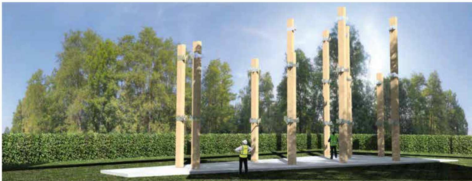
FIRST DAY Tracking and installation of the pillars with brackets
