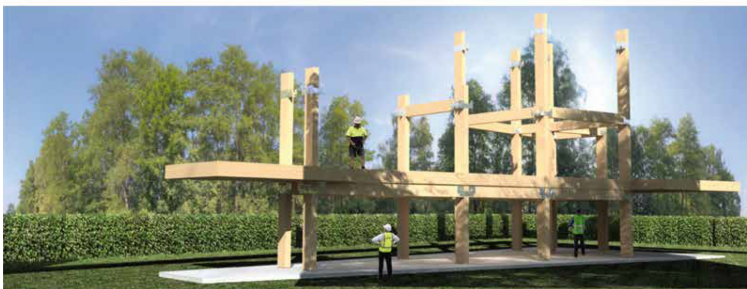
SECOND DAY Installation of the first crowing timber-beams and pillars
